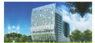
IT Twin Towers Sector 66-A, Mohali
